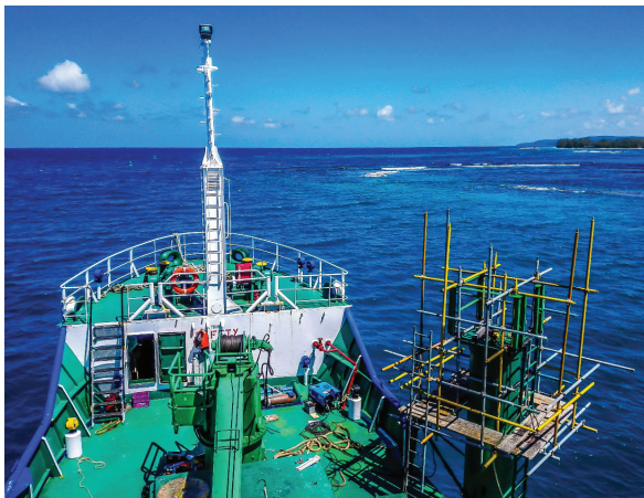
The buoy tender vessel MV Jamaica II assisting with the repair of the No. 7 navigational beacon at Falmouth
